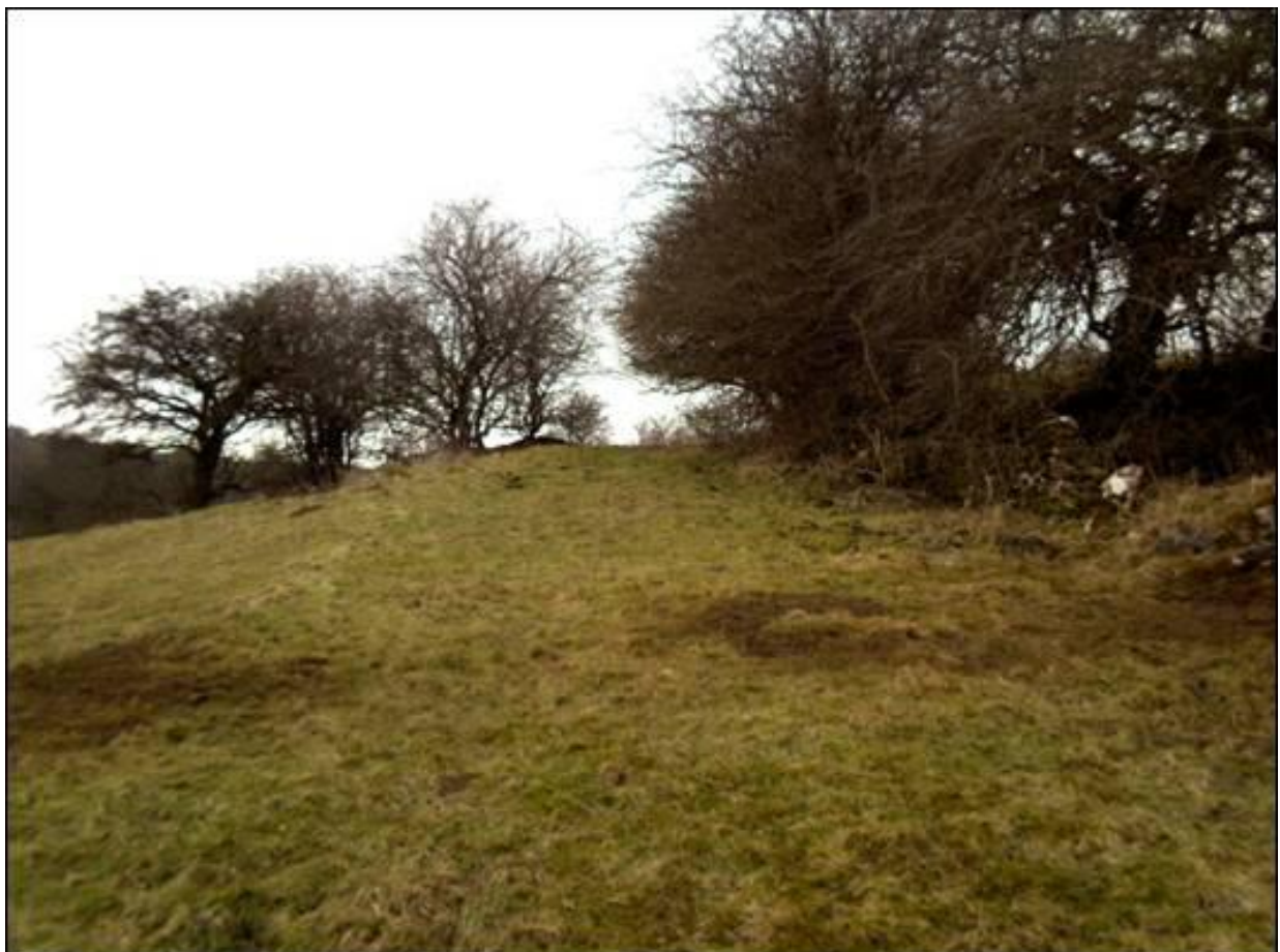
The road formation looking southwards near Grangemill, the terrace clearly falls to the left
