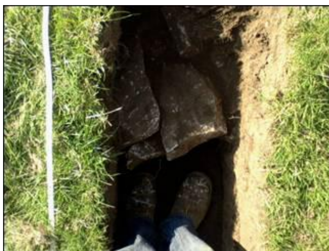
Large edging stones "pitching" supporting the terracing
