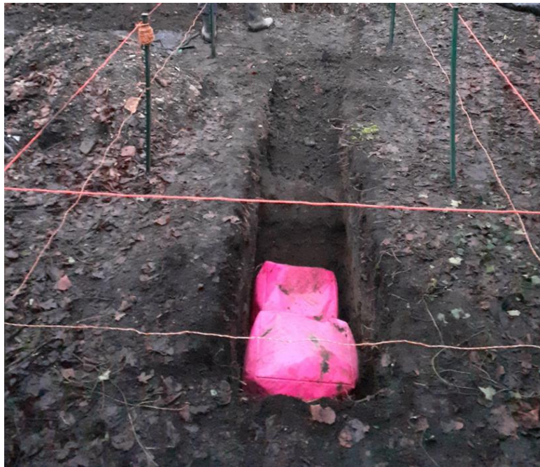
The ditch trench being dug out.
