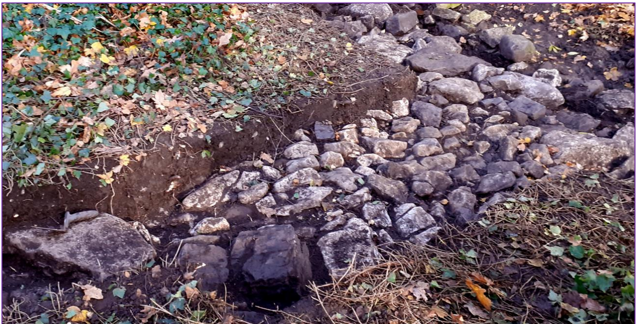
Yard/path? Surface with newly cleared edge of large stones on the left of the picture.
