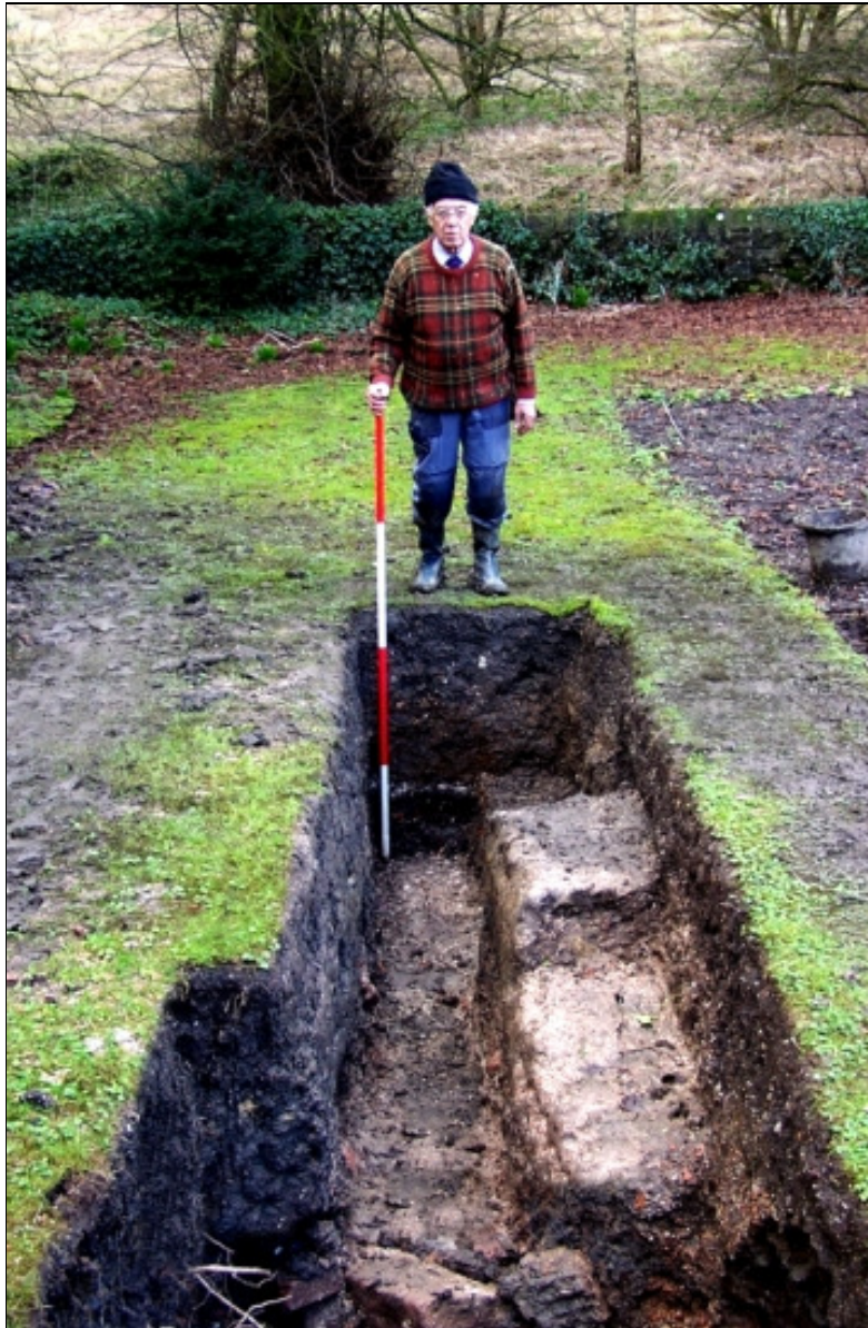
W end of section trench in progress showing depth of mid grey clay layer
