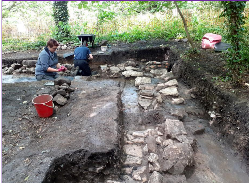
The site showing the north wall foundations of the building, looking west on the 31 st July.
