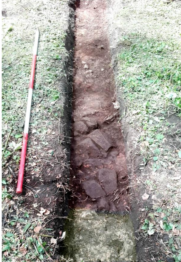
Section Trench looking north: the “widening” appears as grey limestone chatter at the bottom of the photograph at the joint of the pink gritstone of the main road edge.
