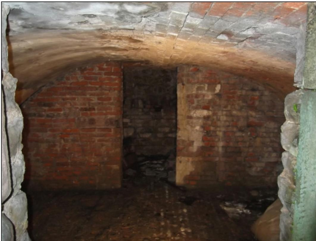
The outer chamber approx 5 metres square and 2 metres high to the top of the brick barrel vault. The floor is also brick, looking north.
